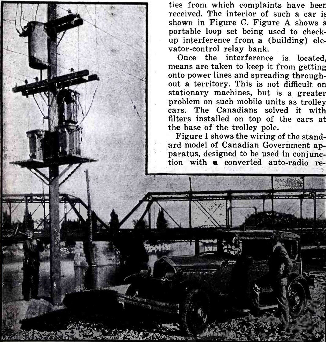
Fig. B. While the "Interference Detective" listens by means of a pair of phones (or loudspeaker, in later models), linesman hits pole suspected of holding defective units. Vibration increases noise.
